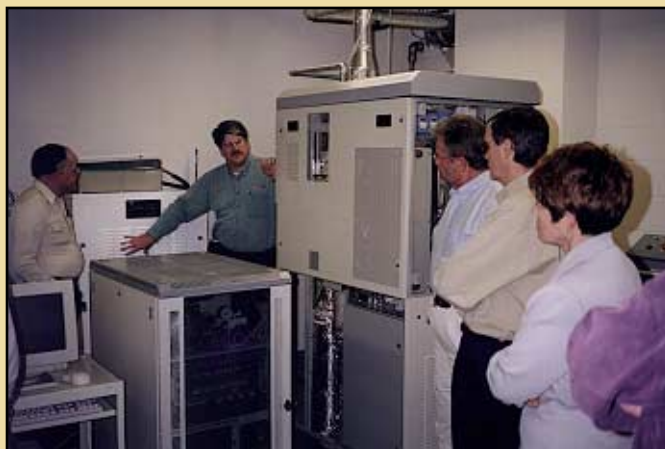
Rural cooperatives such as Delta-Montrose in Colorado are leading the way with the installation of a 10 kilowatt propane-powered fuel cell system. Photo courtesy DMEA
