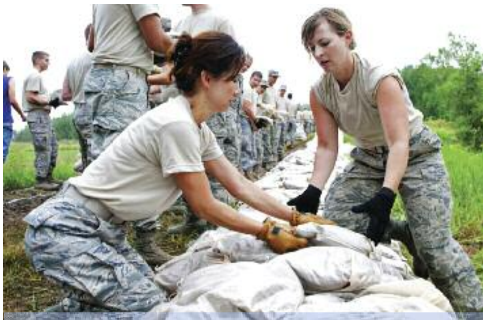
Members of the North Dakota Air National Guard build a sandbag wall to protect a home along the Missouri River near Bismarck, N.D., in June. More than 1,300 North Dakota National Guardsmen worked in the Bismarck-Mandan area to help hold back flood waters. Below: Streets in many towns in North Dakota and Iowa were turned into streams by the flood. Air Force Photos by Tech. Sgt. Oscar Sanchez
