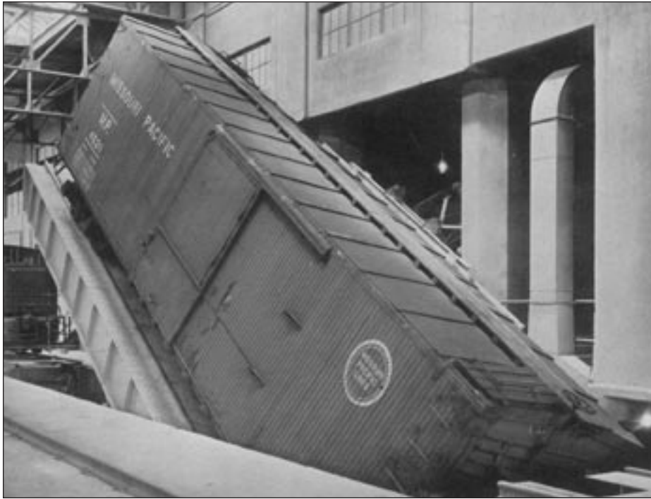
Unloading 1,500 bushels of wheat from a box car only took five to seven minutes and the service of two men at a major co-op terminal in the early 1930s, thanks to up-to-date unloading equipment.
