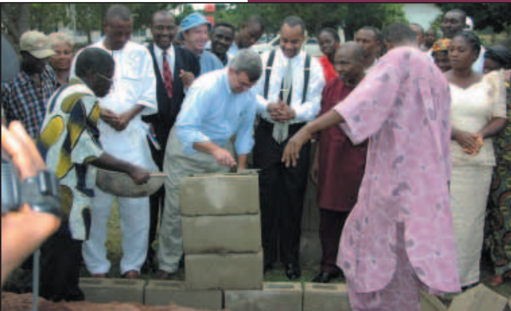
Jeff Jobe, co-op development specialist for USDA Rural Development in Iowa, takes a turn laying the foundation for the new Abia State Agricultural Business Development and Planning Center in Umhahia, Nigeria. USDA is supporting the center.
