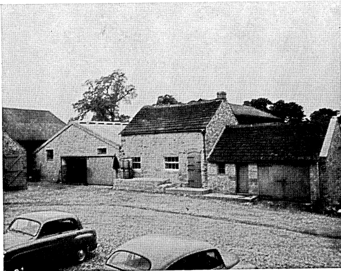
Plate 12: New cowhouse and dairy conversion, viewed from the east.
