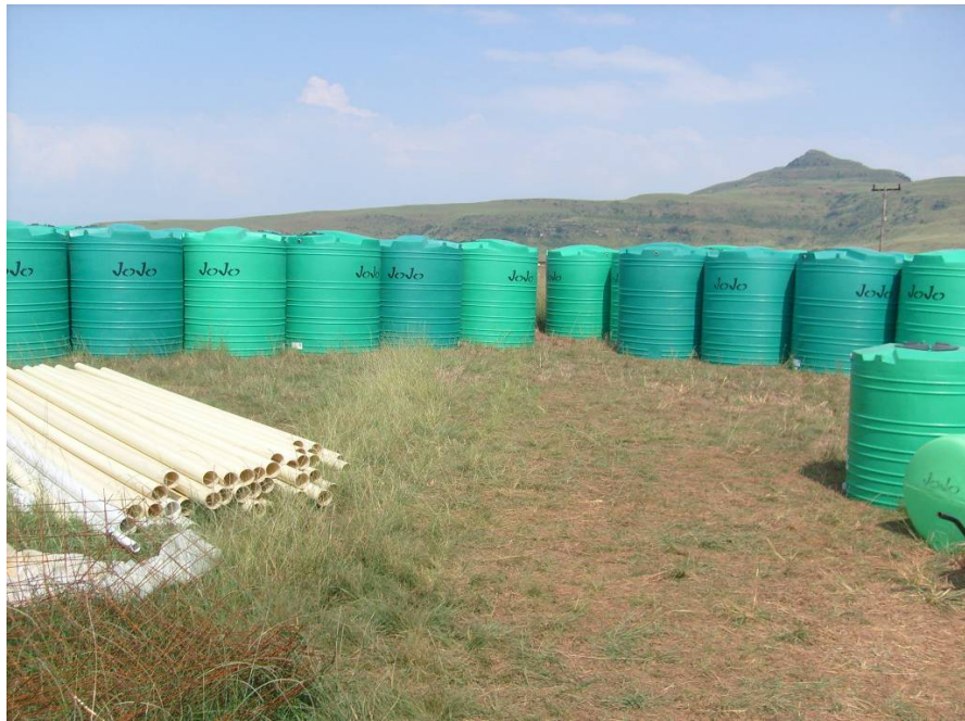
Figure 3.27: More tanks awaiting to be installed in Potshini.
