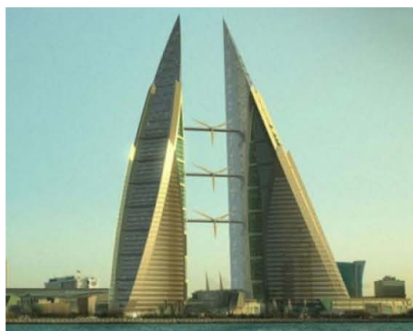
The Bahrain World Trade Center with 3 Wind Turbines
