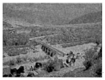
FIG. 5. Inverted siphon and mouth of tunnel 'Kazerun'.
