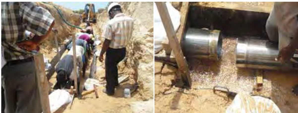
Figure 11.2.8. Installation of laterals (Elongated parallel to the beach line).
