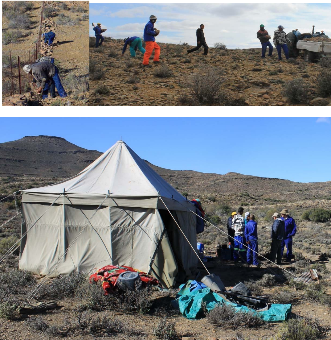
Figure 1: Workers packing rocks along the base of a jackal-proof fence (top left); collecting rocks (top right); and meeting with Piet Gouws and Josef le Roes (a Koups farmer) at a fence team camp site on Le Roes's farm.
