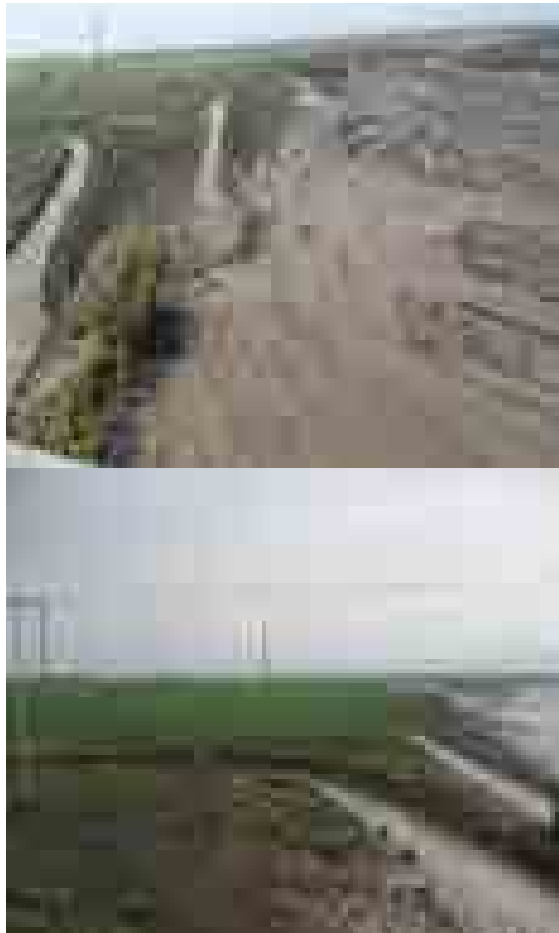
Figure 9.6. The Harosha traditional sbate system having many diversion points along the wadi immediately downstream of a bridge (Eyasu et al. 2012).
