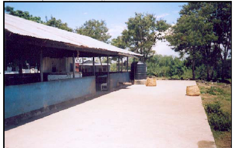
Landing/holding facility with potable water, cement floor
