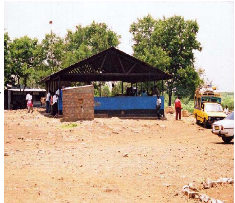
Landing facility with pit latrine, wall, roof
