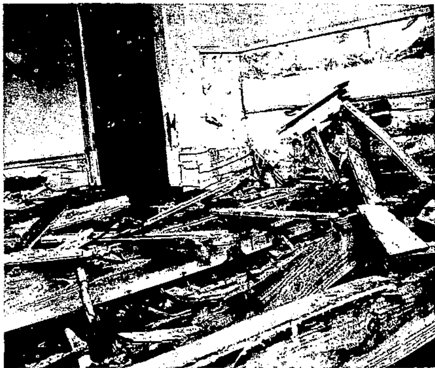
Figure 5.—Framing, flooring, joists, and trim of house decayed by Poria incrassata .
