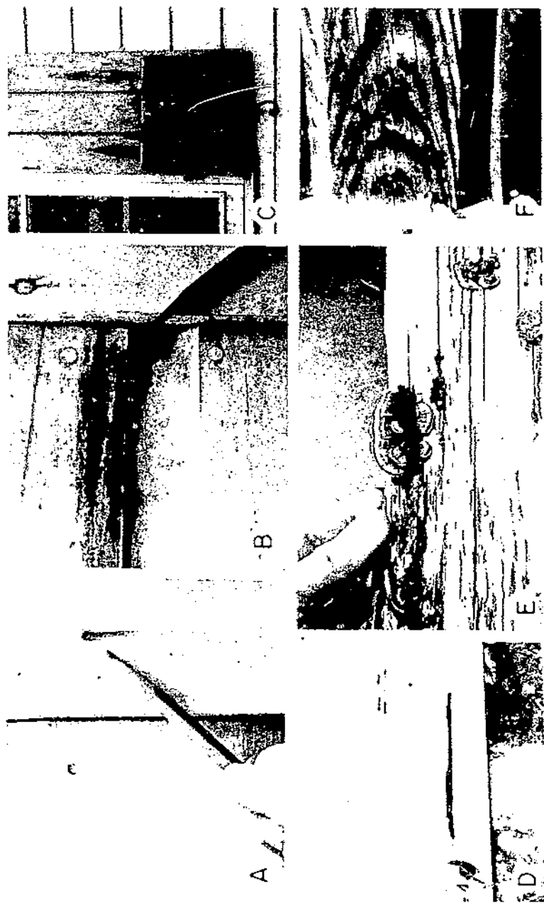
FIGURE 1. Rain seepage may be indicated by: A , Nail rusting; B , fungus stain coming through paint; C , paint peeling, particularly at joints; D , actual decay; E , fruiting bodies of decay fungi; or F , warping of siding and nail pulling.
