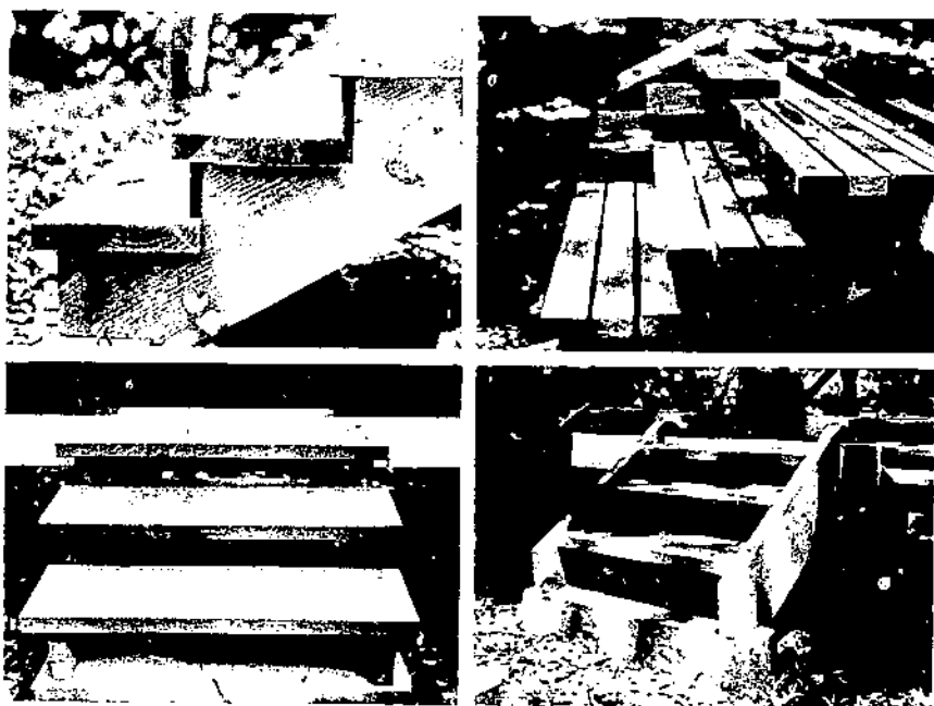
FIGURE 6. Different step designs included conventional carriages with and without risers, solid and split treads, and cleated carriages.
