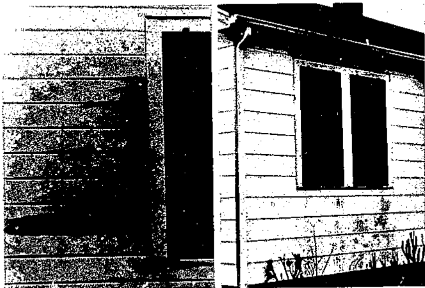
FIGURE 5.—Deterioration of siding on a house 3 years after construction in St. Petersburg, Fla. (left). Shortly after this picture was taken the siding was covered with asbestos cement. Fifteen years later the building was still in good condition (right).
