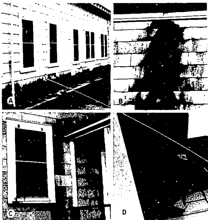
FIGURE 2. Decay associated with roof runoff: A , Splash from sidewalk wetted sheathing and plate at the base of the wall (shingles siding broken for inspection of sill); B , leaks in the horizontal joints of gravel stops are common; C , water from the roof runs down wall and wets window trim; D , sheathing decayed at roof edge when unprotected by a metal flashing.
