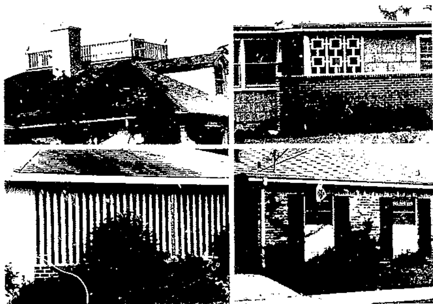
FIGURE 3. Structural members protruding beyond the roof or otherwise exposed to decay-resistant material: A , Columns with high seepage hazard above door; B , rafters exposed to weath; C , church arches exposed to rainwetting; D , roof timbers protruding.
