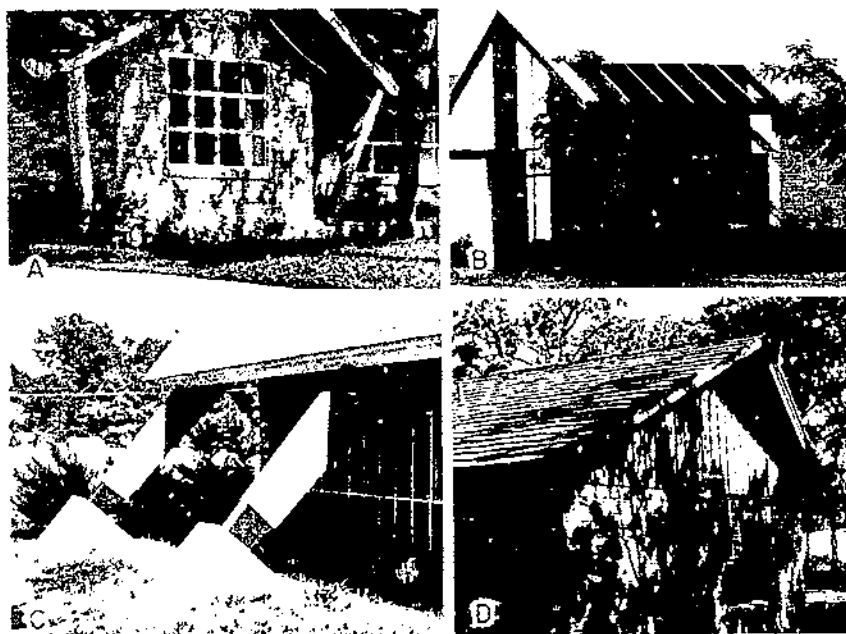
FIGURE 3. Structural members protruding beyond the roof or otherwise exposed to decay-resistant material: A , Columns with high seepage hazard above door; B , rafters exposed to weath; C , church arches exposed to rainwetting; D , roof timbers protruding.
