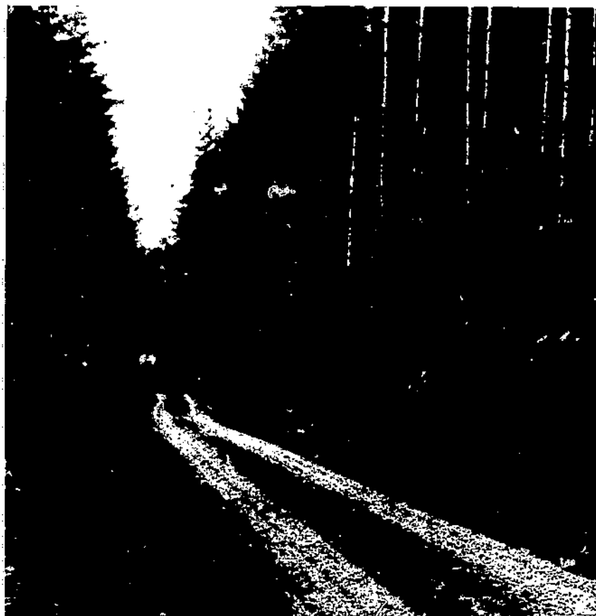
FIGURE 32.—Roads built for thinning should be constructed to serve for the balance of the rotation and for final harvest. They should be adequately drained, well aligned, and graded. This 16-foot road plus ditch and clearing allowance is on the Voight Creek Experimental Forest.
