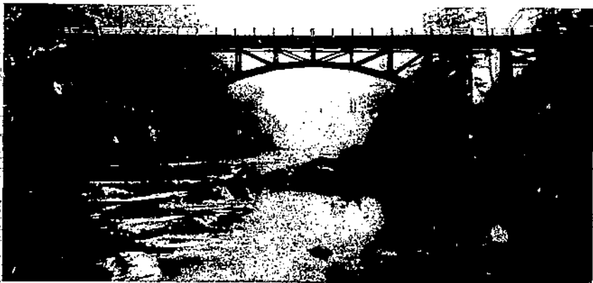
FIGURE 6.— A , Pony truss bridge over Johnson Creek, Multnomah County, Oreg. (span, 60 feet); B , Buffalo Creek bridge at Lewisburg, Pa. (two low-truss, 91\frac{1}{2} -foot spans); C , three-hinged arch bridge in Umpqua National Forest, Oreg. (span, 135 feet).
