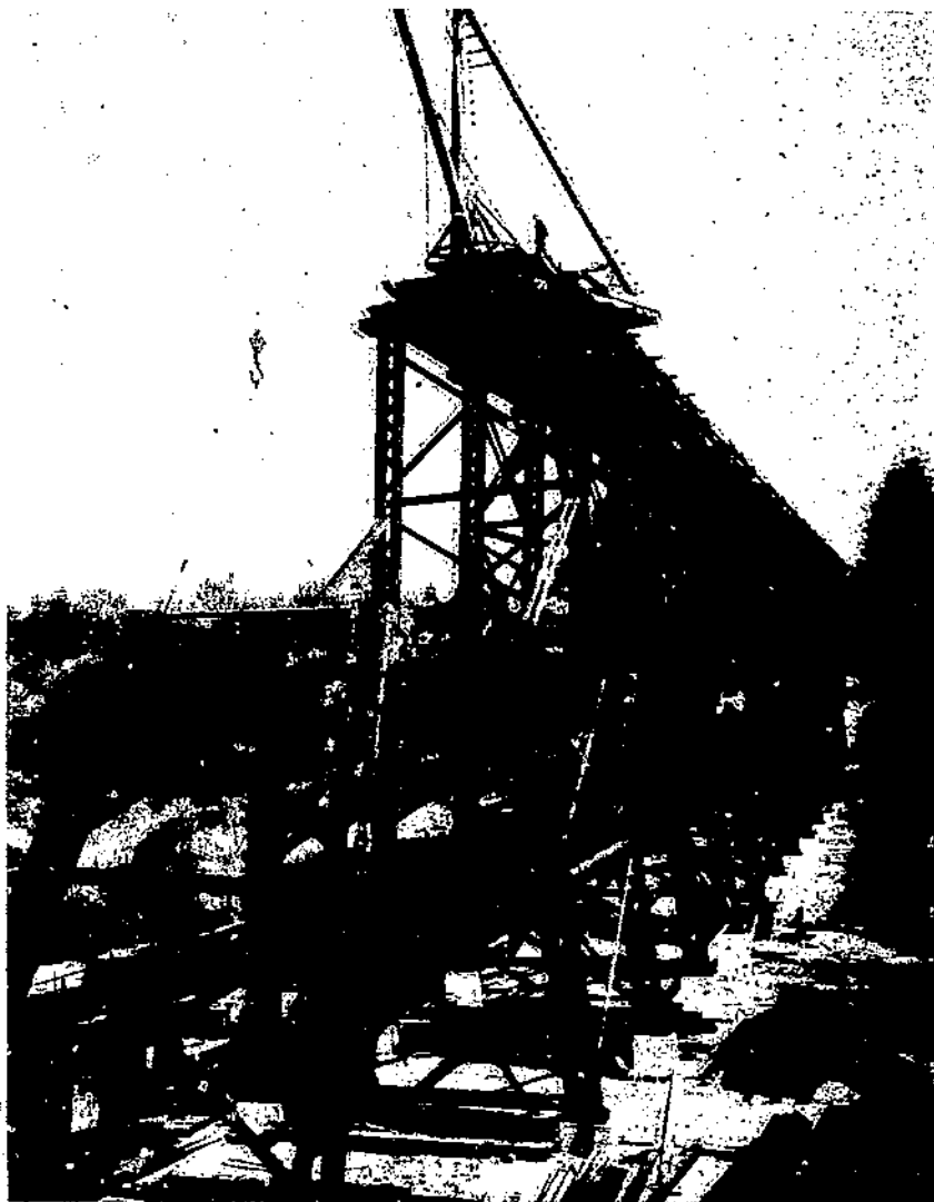
FIGURE 7.—Composite trestle-type highway bridge at Port Angeles, Wash. (length, 755 feet; maximum height, 100 feet).
