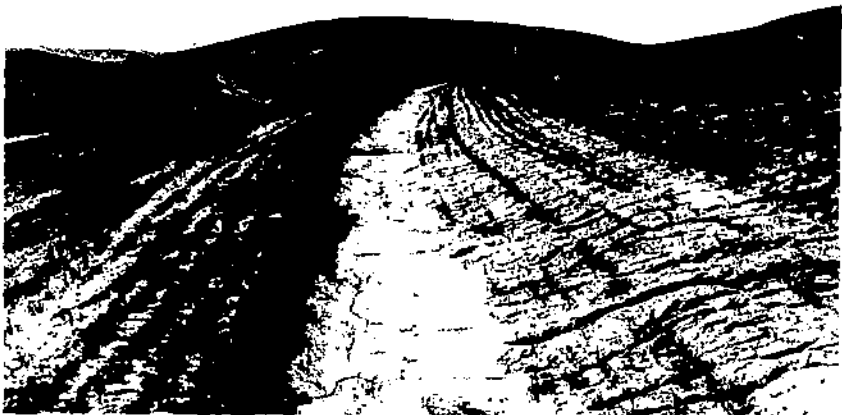
FIGURE 26. Channel of terrace 18, fall of 6 inches per 100 feet, April 27, 1932.
