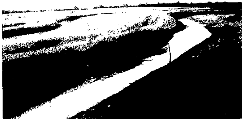
FIGURE 27. Water impounded by closed-end level terraces on heavy compact clay soil.
