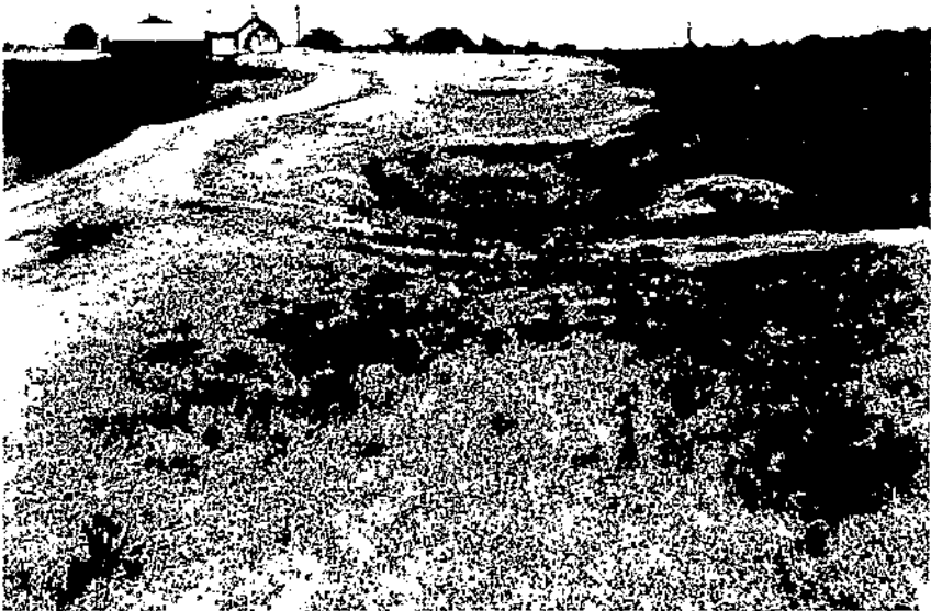
FIGURE 32. Terrace-outlet ditch after Bermuda grass had become established between creosoted plank baffles.
