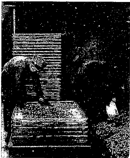
FIGURE 9.—Loading kiln trays with jack pine cones.
