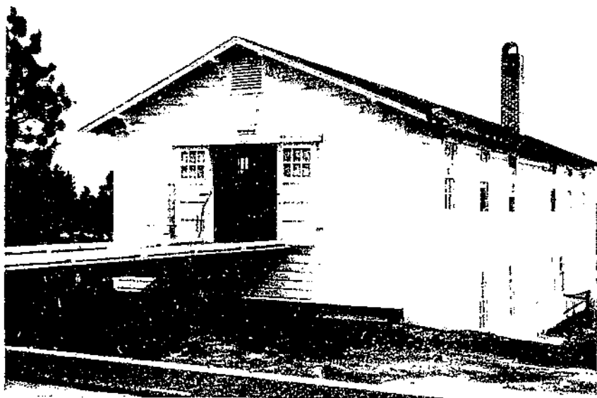
FIGURE 15. Extractory building at the W. W. Ashe Nursery, Brooklyn, Miss.
