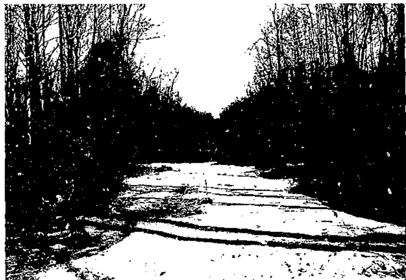
A, Progressive abandonment of bottom land at head of plugged, back-filling Wells ditch near Range WG-6, West Goose Valley, 4 miles west of Oxford, Miss. The ditch, which appears as a broad white line extending from right to left, is completely filled at the left, and the swampy, wooded bottom land appears as a dark area; in the center are three recently abandoned fields, with dark clumps of brush scattered among fresh sand splays; at the right, where the ditch is still partly effective, the light areas of regular shape are cultivated fields. (Aerial photograph by courtesy U. S. Army Engineers). B, View down completely filled drainage ditch at Range WG-6, within the area shown in A.
