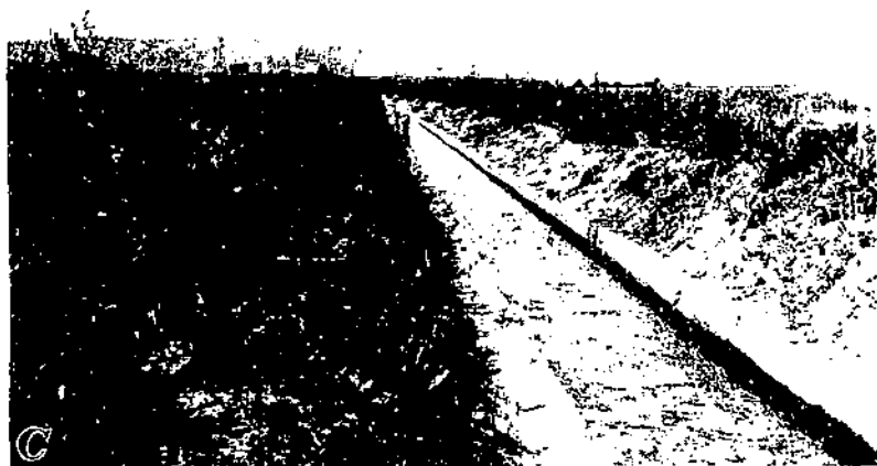
A, Modesto irrigation district main canal, California (No. 99; upstream from station 3 plus 64, on meter bridge.) B, Santa Ana and Orange canal, Calif. (No. 92; upstream from station 12.) Note deposit below highwater line. C, Arroyo Ditch, Calif. (No. 122; upstream from station 8.)
