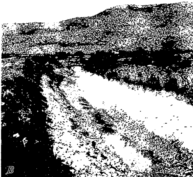
1. A very rough and porous cut in lava rock is made smooth on the bottom by a concrete lining while the sides are made watertight and uniformly smoother than before, with shot concrete. A good place to use Horton's formula for exact sections with different foot and side characteristics. (Division of Reclamation photograph.) B. Cross-sectional, Broken Copper Co., Chile. (Nos. 39 to 50, inclusive.) Cobblestones are more in evidence on this cut than on cuts in western United States that develop a cobble bottom. (Other views submitted by the company showed large crews of men removing the loose cobbles from the bed with a skip and hoist. Note that values of n above 0.000 predominate. View by courtesy of Broken Copper Co.)
