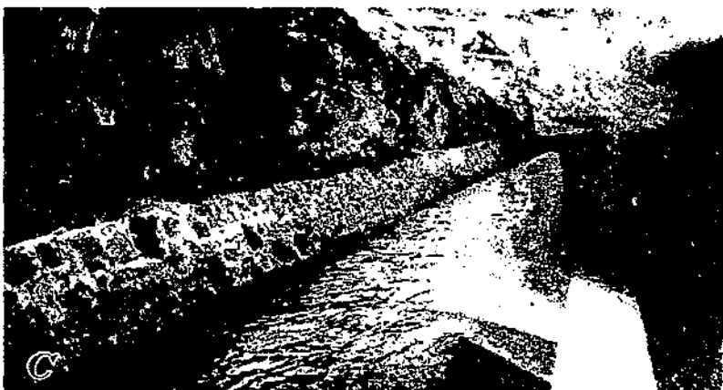
1. Drum canal, Pacific Gas & Electric Co., California. (No. 126.) Lower bank lined with concrete "plank," placed and fixed where needed to prevent erosion. B. South canal, near Auburn, Calif. (No. 98.) downstream from about station 7 plus 20. Many sharp bends. Note highest velocity on inside curve. Water on outside banks up and is inert in direction. C. Deschutes municipal district, near Bend, Oreg. (No. 128.) downstream from station 2. Masonry walls and concrete floor.
