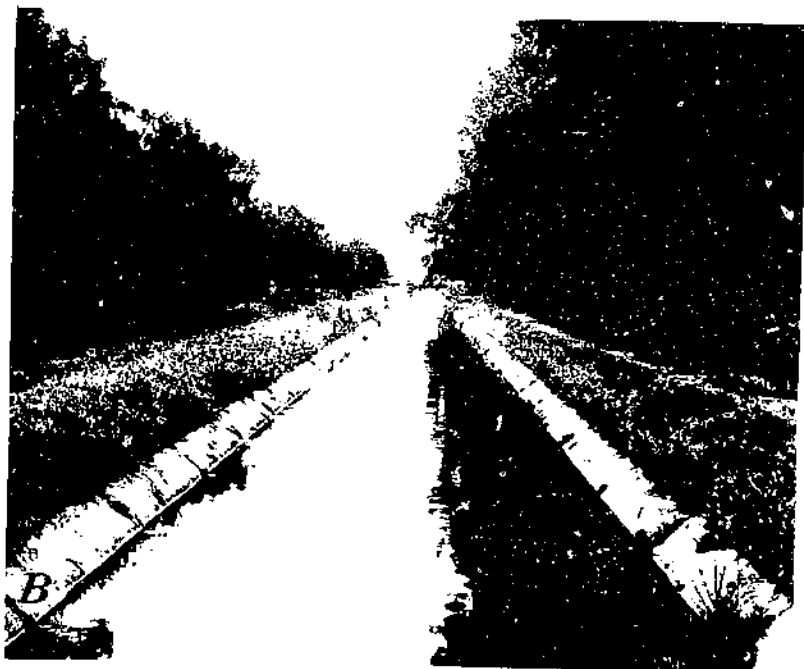
1. Main canal, Kittitas division, Yakima project, Washington. (Constructed about 1929. Excellent example of concrete poured behind screeding and standing platform. Designed with p = 0.014 ; the actual value was about 0.013 of less. Same 615 second-foot of water was in canal when photographed. A , A lateral in California, lined more than 20 years before the picture was taken. Low velocity of warm, clear water conducive to aquatic growths. Note weeds growing in expansion joint cracks. Bureau of Reclamation photographs.
