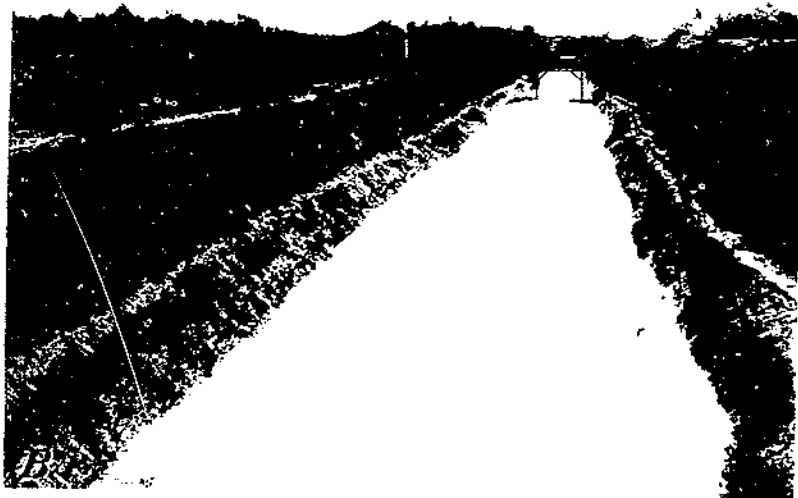
1. A new canal conveying clear water. The original trapezoidal shape beginning to round off at the corners to form the eventual ellipse (with nearly vertical sides if grasses root along the bank). B, A new canal or one recently cleaned, conveying silty waters. The mud berms develop at the sides and crowd in until an approximation to a regime channel is reached. Sometimes these berms are 2 feet or more wide while not more than a tenth of a foot or so has deposited on the bottom. Original material erodible at velocities of 3 feet per second becomes protected with a slick coat that will withstand velocities of 5 to 6 feet per second. Photographs from Bureau of Reclamation.
