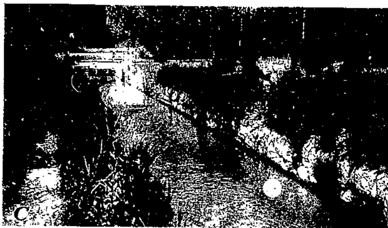
A, Upper canal, Riverside, Calif. (No. 132; upstream from station 2 plus 30.) Note meter station. B, Jacobs ditch, Boise, Idaho. (No. 431; downstream from station 0.) Rubble masonry, smoothly plastered walls, concrete bottom. C, Jacobs ditch, Boise, Idaho. (No. 432; upstream from station 1.) Unclinked rubble sides and bottom.
