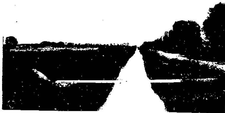
A. Santa Ana and Orange canal, California, just after being cleaned. (No. 257; upstream from station 10.) B. Central main canal, Imperial Valley, near Calexico, Calif. (No. 268; downstream. Portable gaging car shown over station 0.) When inspected in 1938 this reach of canal was completely free of brush and weeds as shown. Modern canal maintenance is conducive to better capacity conditions. C. Beech canal, Imperial irrigation district, California. (No. 315; upstream from meter station 10.) The muddy waters discourage aquatic growth in the water prism, but the fertile silt banks grow dense vegetation that drags down into the water prism and develops a high value of n .
