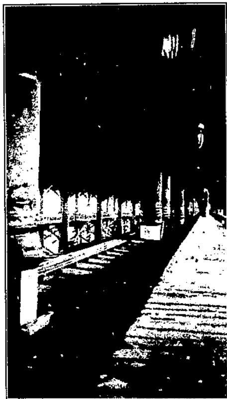
FIGURE 32.- Air doors of Santa Fe precooling system at San Bernardino in place over hatch at each end of car. Air is blown into the car at one end and is drawn out at the other end.
