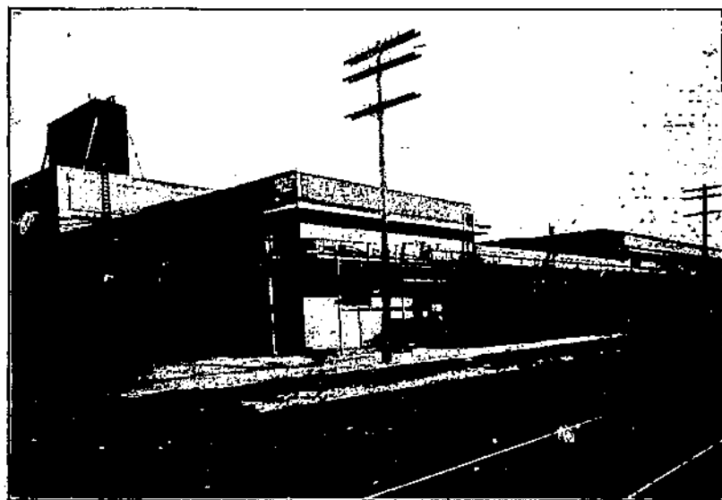
FIGURE 27.—A typical warehouse precooling plant located at the rear of a packing house. Note block-and-tackle arrangement at each end of the first car at left used to lower whole 300-pound cakes of ice into the bunkers.
