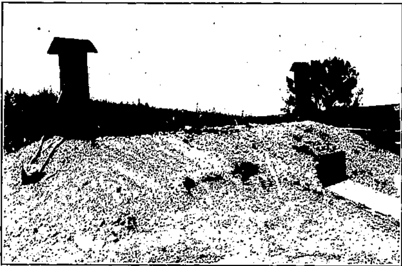
FIGURE 6.—Bee cellar of the dig-out type. This cellar has a dirt floor and plank ventilating shafts. The side walls and top are constructed of logs. More permanent cellars of this type have concrete floors and side walls.
