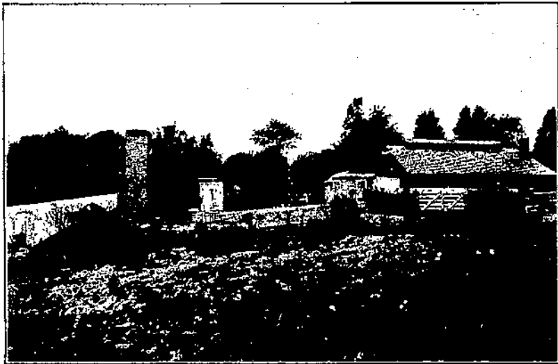
FIGURE 3.—Barn used to house test animals exposed to anthrax; incinerator on the left.
