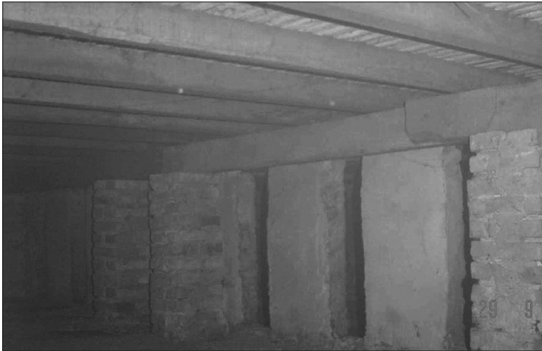
Fig. 6. The under-plenum duct inside the drying bin of an 8 t dryer (“Ong chim” in Vietnamese).
