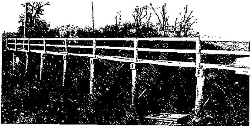
A, Concrete suction bay reinforced by concrete-filled caissons which support rear of pump-house over the bay. Liverpool drainage and levee district. B, Inexpensive suction bay of wooden planks and piling to prevent raving of end of drainage ditch. Big Swan drainage and levee district. C, Trash screen upstream from suction bay supported by substantial wooden trestles. Hunt drainage and levee district.
