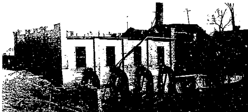
A, Simple brick pump-house. Des Moines-Mississippi drainage and levee district. B, Metal pump-house on reinforced concrete foundation carried above pumping floor; also well-designed trash screen. Lacey, Langeller, and West Mantanzas drainage and levee district. C, Low-cost pump-house of concrete blocks. McCre Creek drainage and levee district.
