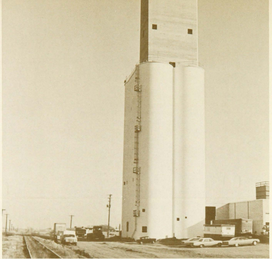
This subterminal elevator was being constructed last summer and fall in Madelia. A subterminal can be defined as an elevator which purchases more than half its grain from other elevators. Subterminals can be a sales outlet for country elevators which don't want to make multiple-car shipments.
