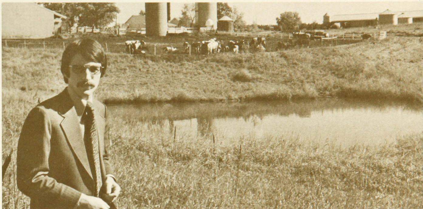
Stephen Ziegler inspects a runoff control system on a Washington County dairy farm. Runoff from the exposed lot is funnelled by a diversion channel through a settling basin to the holding pond. Effluent from the holding pond is periodically irrigated onto cropland or pasture.
