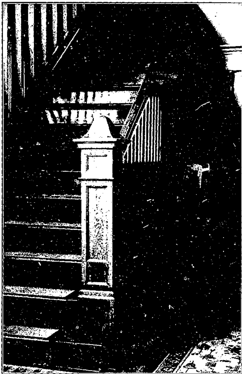
FIGURE 22.—Western larch stairway and panel strips showing effect obtainable with natural and stain finishes
