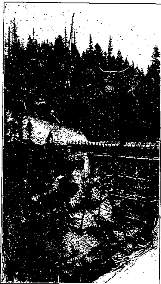
FIGURE 28.—A highway bridge of western larch. The strength and moderate decay resistance of western larch make it a desirable species for bridge timbers
