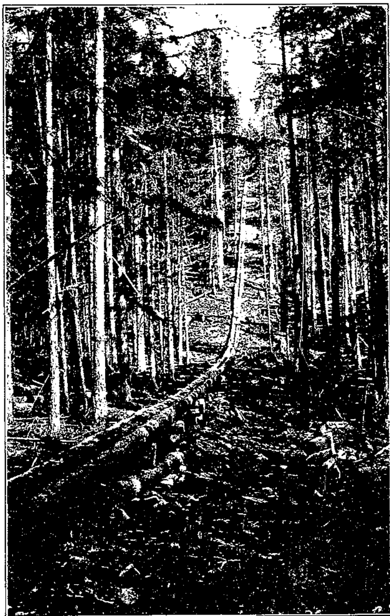
FIGURE 30.—A logging chute constructed of larch fir. The high degree of hardness and decay resistance of western larch adapt it to such outdoor uses where it is in contact with the ground and subject to exceptional loads and heavy wear.
