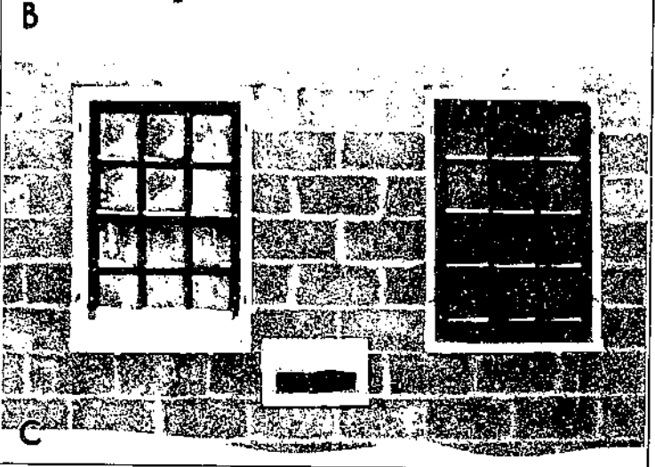
A, View of test barn A-B from the southwest; B, view of test barn C-D from south; C, barn windows with and without storm sash. The window on the right is equipped with storm sash
