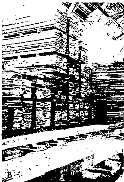
Storage of seasoned lumber under shelter. A, The exterior of a storage shed suitable for air-seasoned lumber, showing its open side. B, A part of the interior of the same well-built shed. The lumber is laid flat on stringers, with heavy stokers separating successive piles; additional stringers at the ends of the piles might be better practice than the small number now used.
