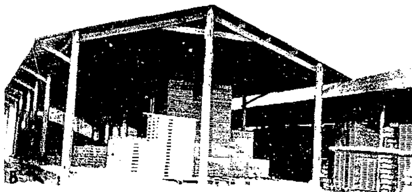
Dimension stock piled for immediate and for ultimate economy: A, Lap-piled flat dimension stock. B, a general view of an open shed sheltering dimension stock during seasoning
