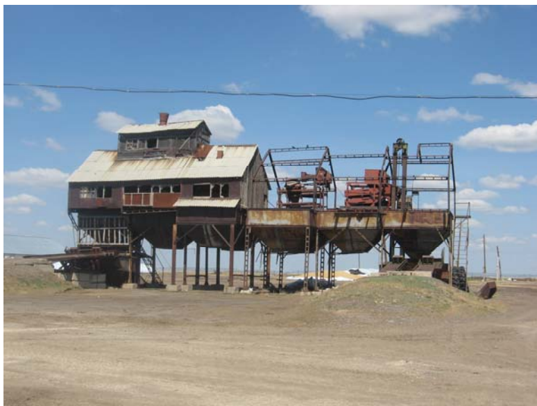
Picture 2: Obsolete grain storage
