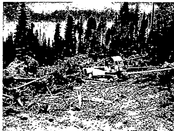
Figure 22.—Mechanical scarification using a brush blade mounted on a bulldozer, Kootenai National Forest. Logging slash and brush are pushed into piles or windrows and burned.
