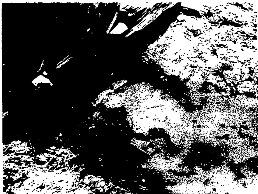
FIGURE 10.—Irrigation canal oiled to form a barrier. Two barrels of oil are in position. When one barrel is emptied by the steady release of a small stream of oil, the second is ready for immediate use.
