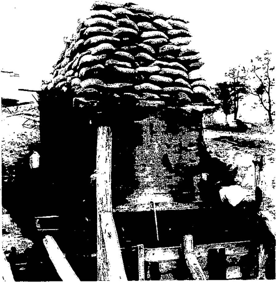
FIGURE 3.—Casing weighted with sand bags to facilitate lowering in partly excavated trench.
