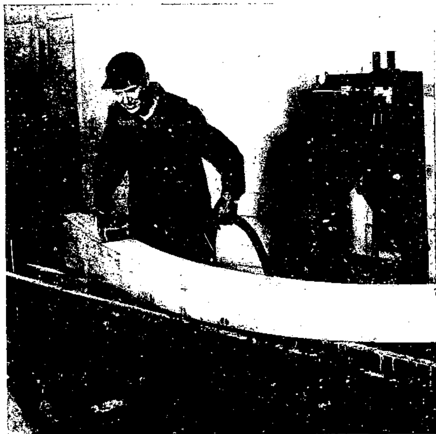
FIGURE 41.—Portable planer used for surfacing straight or curved timbers.
