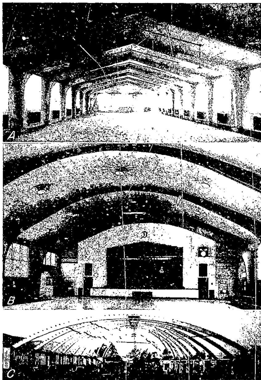
FIGURE 1.—A, Laminated arches span 46-foot-wide service building at Forest Products Laboratory; B, laminated arches of 63-foot span in high school gymnasium at Darlington, Wis.; C, laminated arches of varying span and shape for theater at Los Angeles, Calif.
