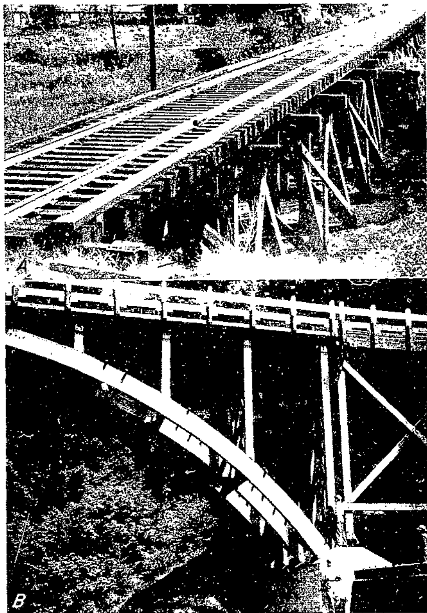
FIG. 10. A , Railway trestle of laminated southern yellow pine timbers; stringers, posts, and caps glued with intermediate-temperature-setting phenol-resorcinol resin and pressure-treated with creosote. B , Loom Lake bridge, in Oregon, supported by four 103-foot-span glued laminated arches; inner members 11 by 24 1/2 inches in cross-section, outer members 9 by 21 1/2 inches in cross-section; members glued with phenol-resorcinol, laminations pressure-treated with Wolman salt before gluing.
