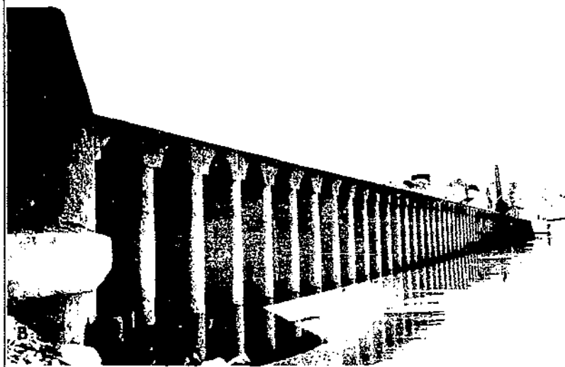
A. Rockwood heading, intake of main Imperial Valley canal from Colorado River (showing suction dredgers removing silt) B. View of Rockwood heading from the Colorado River
