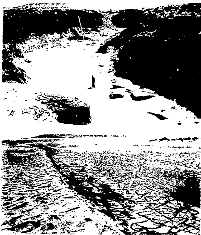
FIGURE 8.—A, View from 1936 of E. J. O'Connell, 35-foot-long arroyo cut by runoff from 45,000 acres, with the spillway structure in background; B, View from same angle in 1947 from flood plain.
