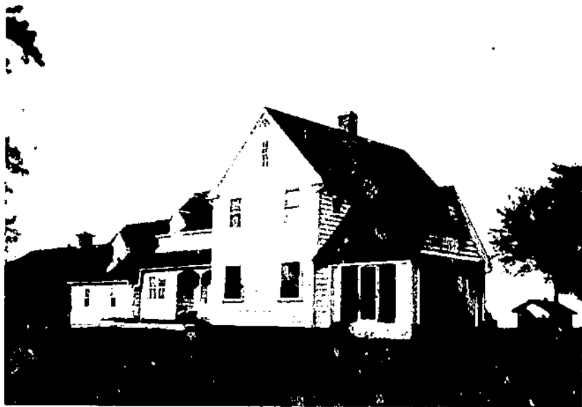
FIGURE 35.--House No. 7-R from the southwest.
