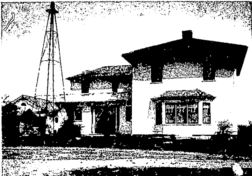
FIGURE 41.—House No. 8-R from the south.
