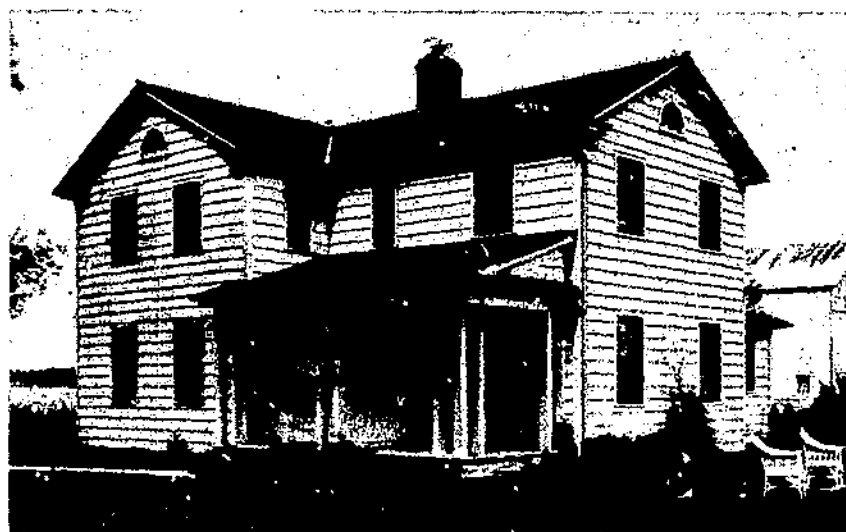
FIGURE 23.—House No. 5-R from the southwest.
