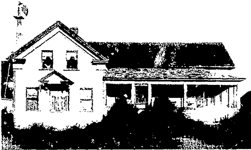
FIGURE 7 - House No. 2 from the west.
