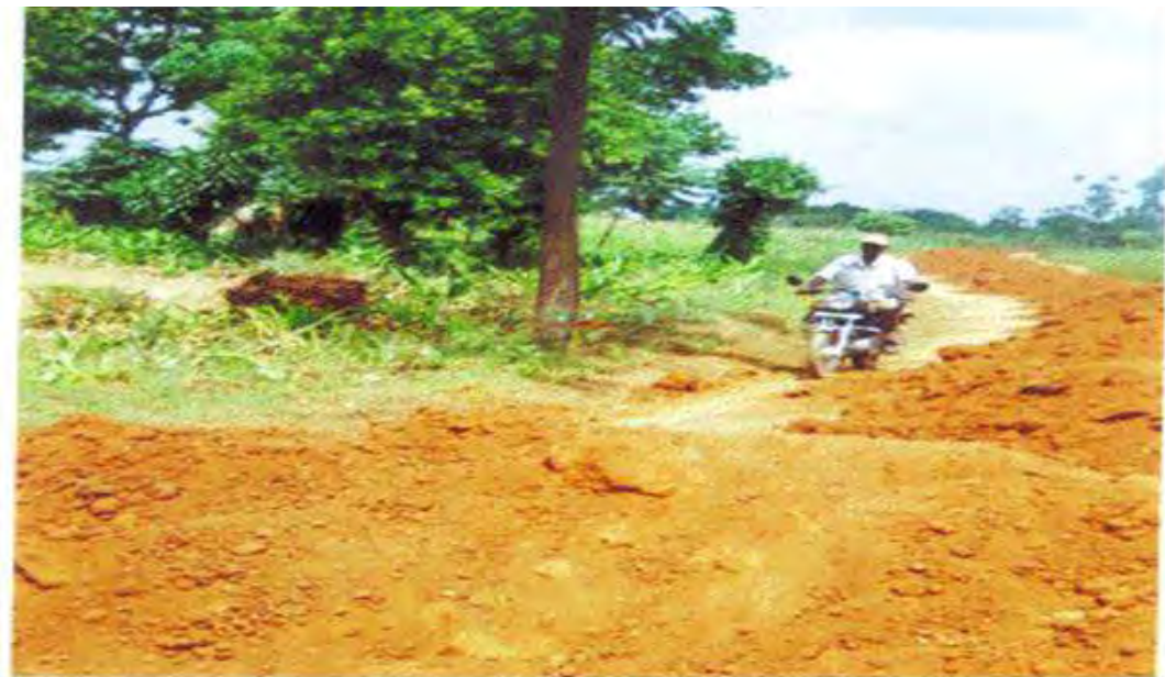
Figure 3: Unspread and Overstayed Murrum on Kachocho Road being Under Rehabilitation
