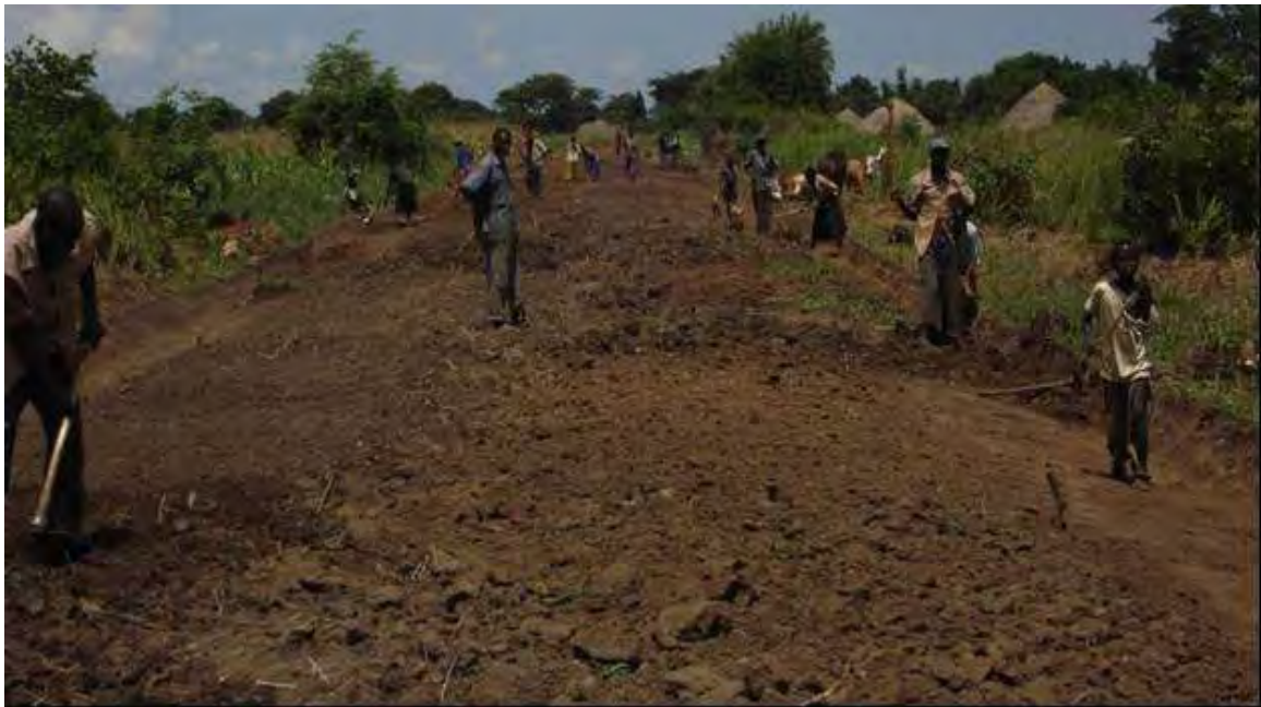
Figure 2: Labour-Based Activities on Apapai-Ogera Road in Serere County, Soroti District
