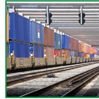
Page 16 Alameda Corridor Transportation Authority
