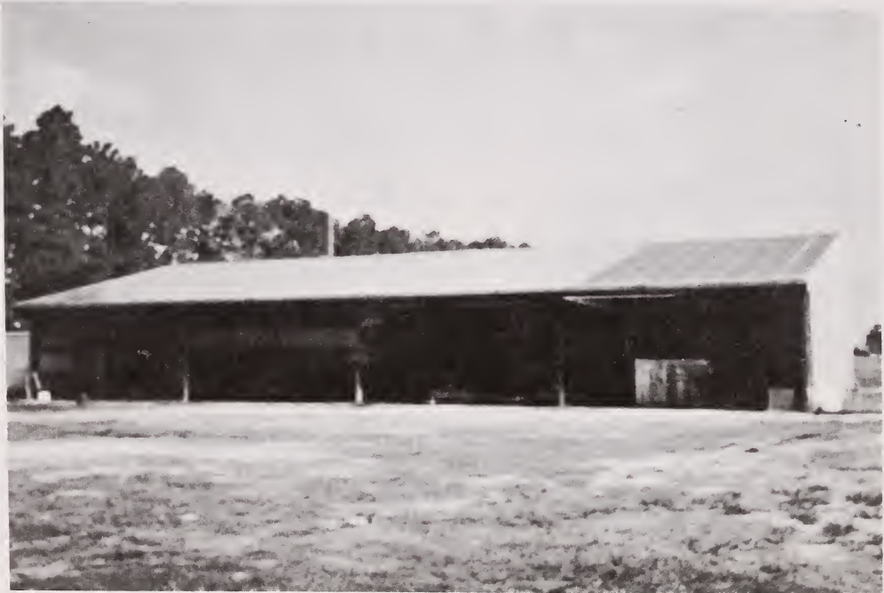
Figure 7--Multiple-use solar curing and drying facility at Tifton, Georgia
