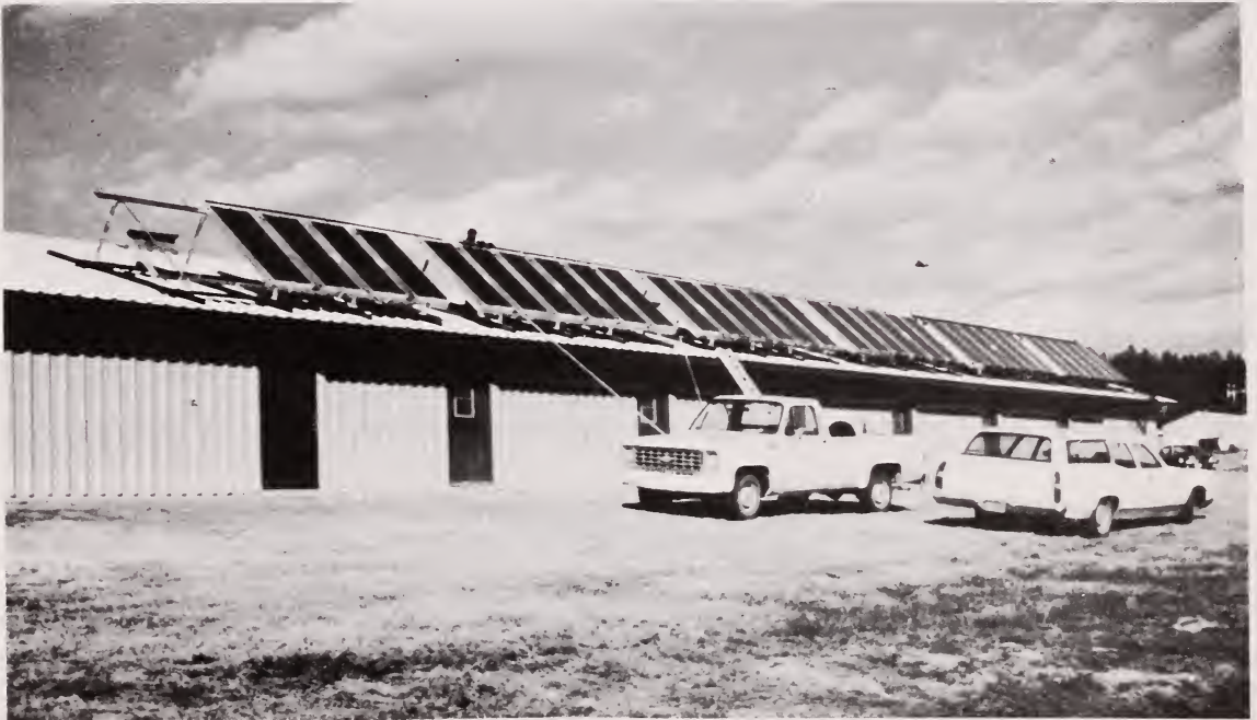
Figure 4--Solar energy research and demonstration facility for broilers at Auburn University showing roof-mounted flat-plate collectors.
