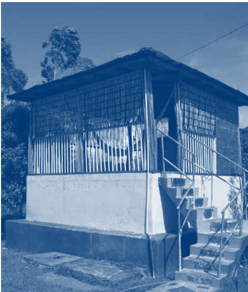
Figure 3.15. An excessively large household storage tank with a bar-discotheque on top in La Palma-Tres Puertas (Source: CPWF-MUS project)
