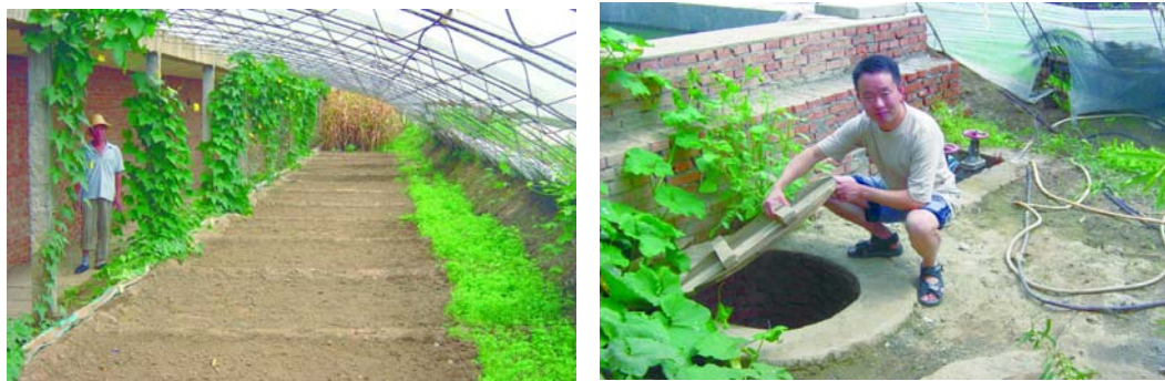
Figure 7. (left) Poly-greenhouses with FILTER plots, underlain with a subsurface drainage system; (right) Cheng Xianjun inspecting the drainage sump into which subsurface FILTER drainage water flows. This drainage water (with pollutants reduced below EPA limits) could be reused, or discharged into surface water bodies.
