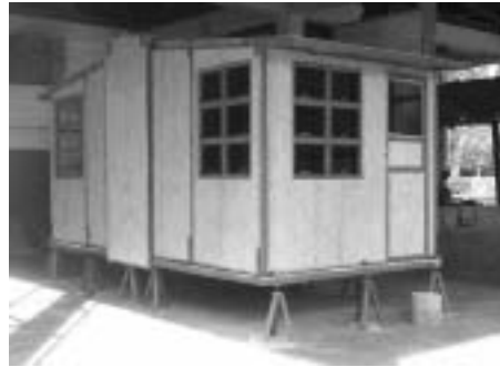
b. The second prototype assembled at the shop. Accessories and stairs are not installed.
