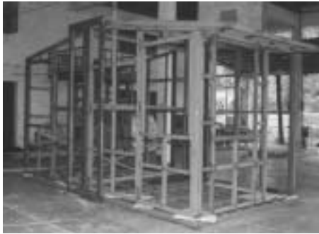
a. Structural frame of the second prototype emergency shelter
