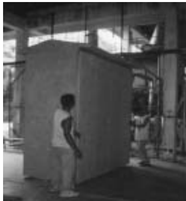
a. Trial fitting of the folded wall, floor and roof components in the case
