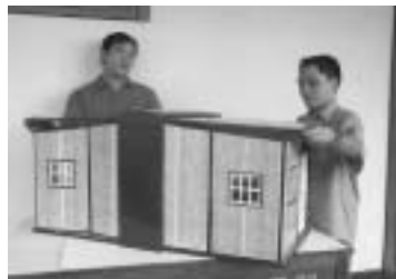
g. The walls are locked in place and the roof temporary supports are removed
