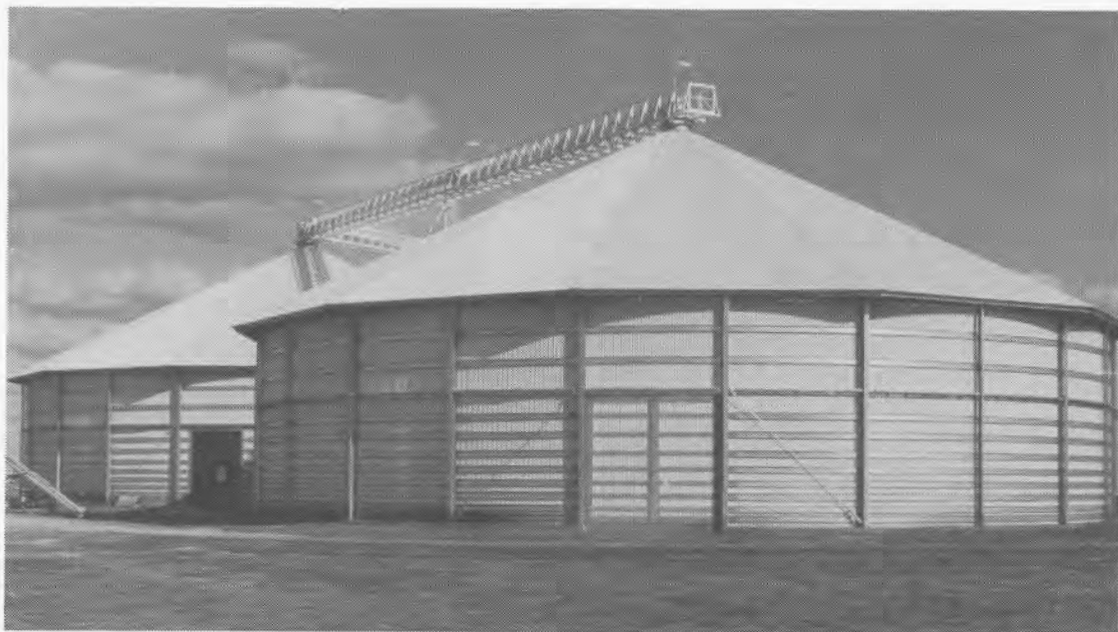
Fig. 9. Gastight bolted light gauge steel silo.
