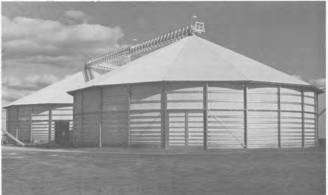
Fig. 4. The 'Safeway' silo, a type of 'squat' grain silo.
