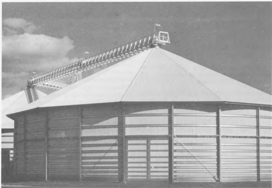
Fig. 2. Large doors allow squat storages to be used for economical, sealed-for-fumigation bag storage when not required for bulk grain, a useful option at a port where bagging is done.
