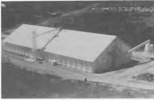
Fig. 2. A typical 60 000 tonne grain shed in Queensland, Australia.
