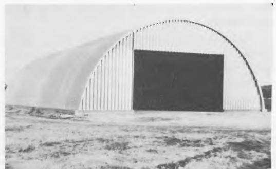
Fig. 7. An arch shed for grain storage, made from deeply corrugated, light-gauge, galvanised steel sheeting.
