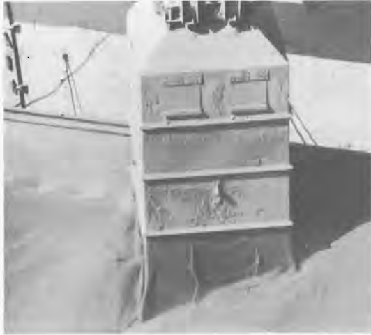
Fig. 5. Dust suppressor at a Cargill Inc. (USA) export terminal, 1982
