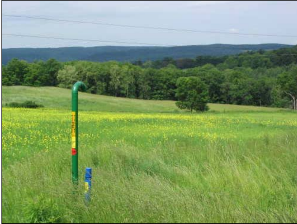
Photo 1. Pipeline marker, Schuyler County, NY.
