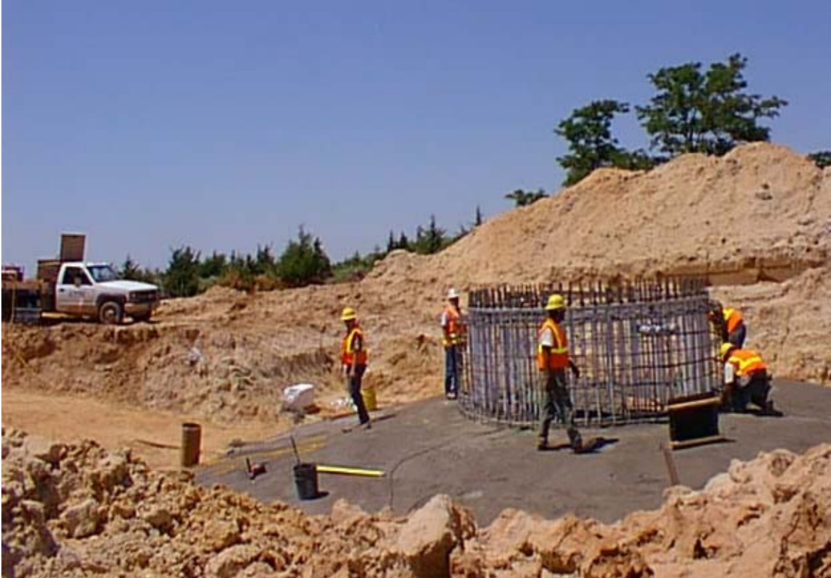
Photo 2. Constructing a wind turbine foundation in Woodward County, Oklahoma (Oklahoma Municipal Power Authority 2003)
