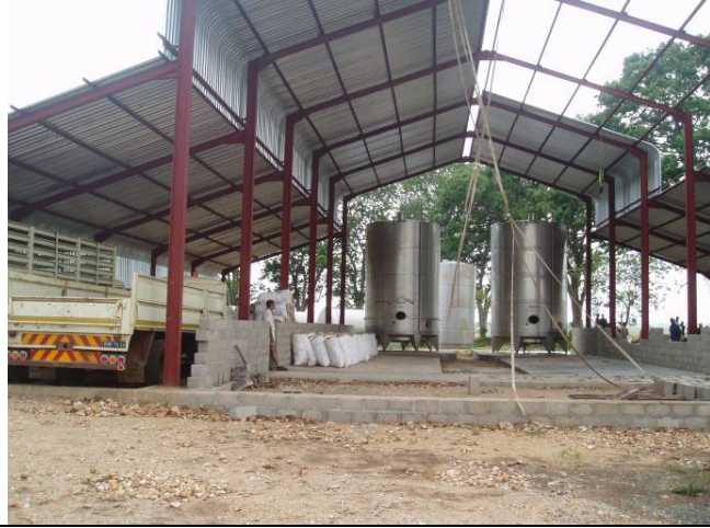
Figure 8. Ethanol Plant under Construction, Mocuba Mozambique
